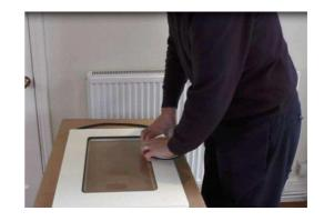
Now you're ready to fit the rubber gasket into place, you'll notice it has a flat edge and a ridged edge. It's the flat edge that fits against the glass, and the ridged edge that faces upwards. Some types of rubber gasket also have a white strip on them, which should face upwards.
