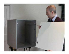
Attach the top hinge first followed by the bottom ones. If the door is heavy, get someone to support the weight of the door while you do this. Once all the doors are attached, refer to our guide on adjusting hinges. See page 26-27.
