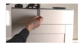
Now we need to calculate where the first handle hole is going to be. Start by measuring the width of the drawer front.
