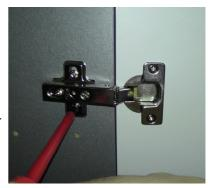
If when you loosen those screws off, the back plate is a little bit stiff, you can just tap the back plate very gently with a hammer and that will loosen it off allowing you to then move the back plate up and down. There is quite a lot of adjustment in the back plate to allow you to do that.
