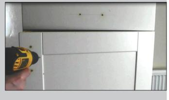
little block of wood behind where the drill hole is going to be so when the drill punctures the back of the door it doesn't damage the surface.
