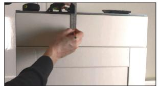
Start by measuring the width of the drawer front
