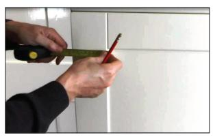
drill a hole 55mm from the top of the door and half way in the centre of the door frame which is 45mm from the edge of the door.
