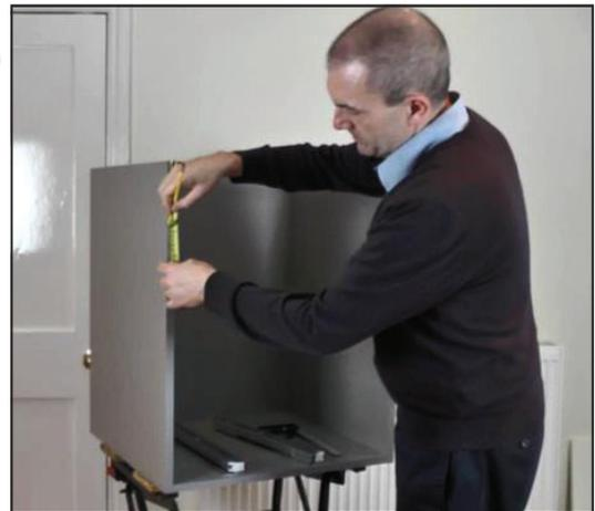
On the drawer runner itself you will see that there are rows of fixing holes. Having decided how far above the bottom of the drawer front the drawer runner is going to sit, draw a pencil line on the front of the unit to show the centre line of those holes. Using a spirit level extend this line from the front to the back of the cabinet. Then draw a vertical line 37mm back from the front of the cabinet - this is where the 3rd hole back on the drawer runner will align
