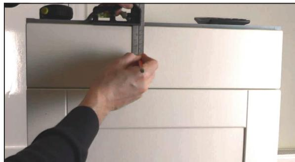
Now we need to calculate how far the first hole is going to be from the edge of the drawer.
