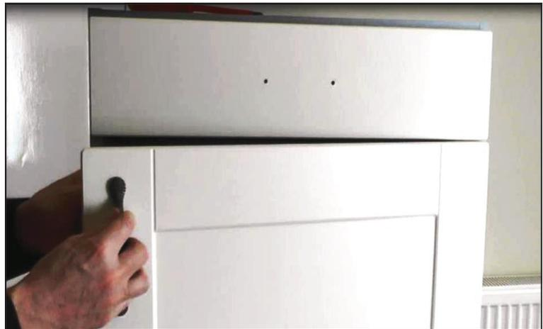
Check that they are level and in the right position. Having the handles level and in the same position so that they line up on every door is the difference between having a job that looks professionally fitted rather than something that is less than good.
