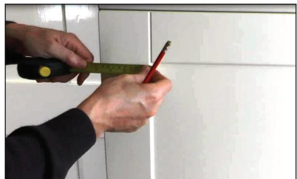
drill a hole 55mm from the top of the door and half way in the centre of the door frame which is 45mm from the edge of the door.
