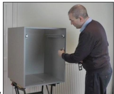
Mark the two fixing holes positions, taking care to ensure that they are at the centre of the backplate screw holes, otherwise you will not have sufficient movement in the backplate should you need to adjust its position later.
