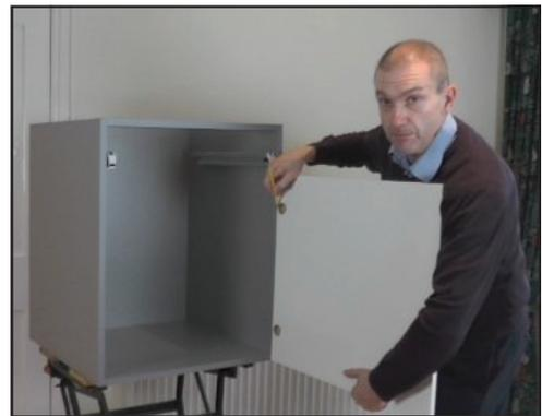
Then draw a second line, a vertical line 37mm from the front of the unit. This line shows the distance from the front of the unit to where the backplate fixing screws will be.
