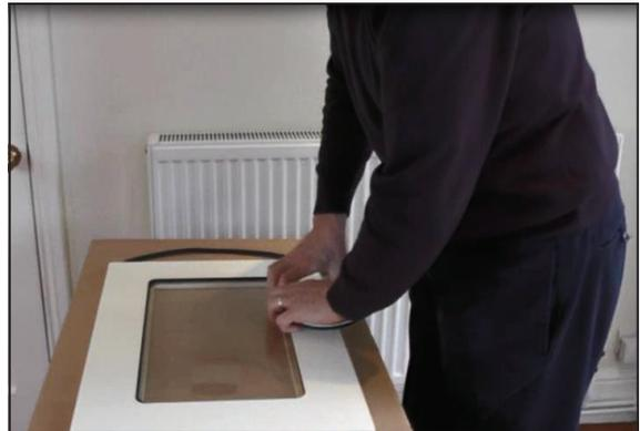
Some examples of rubber gasket have a white strip which should face upwards, but that may change from time to time so if yours doesn't have a white strip on it, just make sure you have got the flat strip against the glass.
